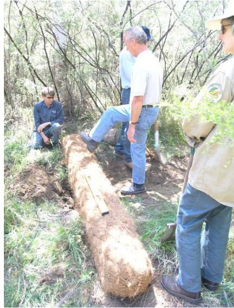
Plate 6-3 - Round Coir Logs Installed to Spread Water
